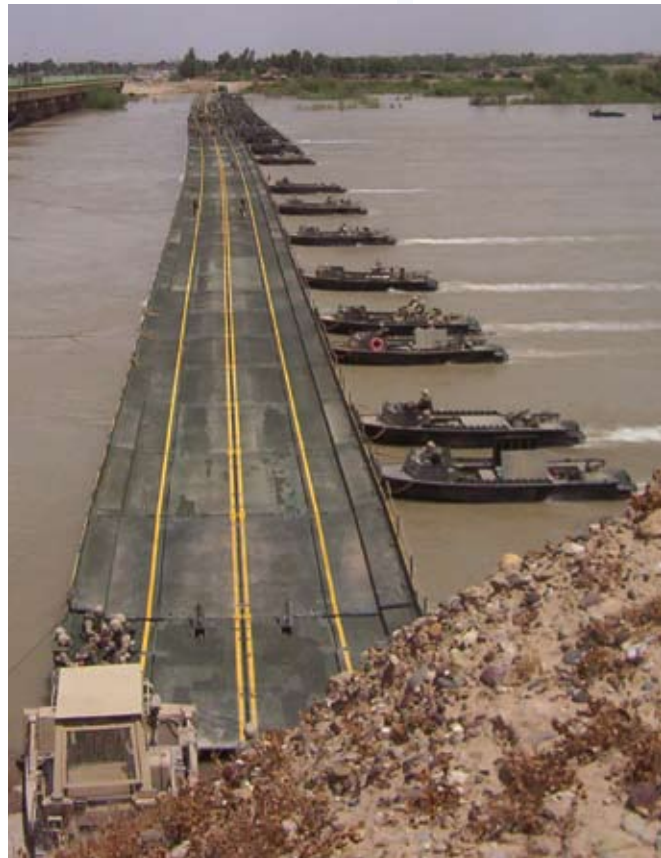
Bridge Erection Boats (BEB) emplace the Improved/Standard Ribbon Bridge sections (above).
